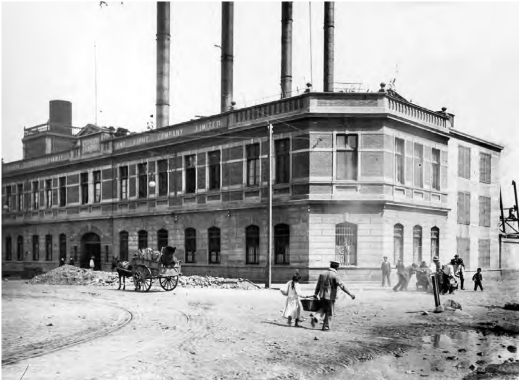
Sanitago: Damages at the main building of the Chilean Electric Tramway and Light Company Limited, Estación Central (Photo: Fritz Sauter)
