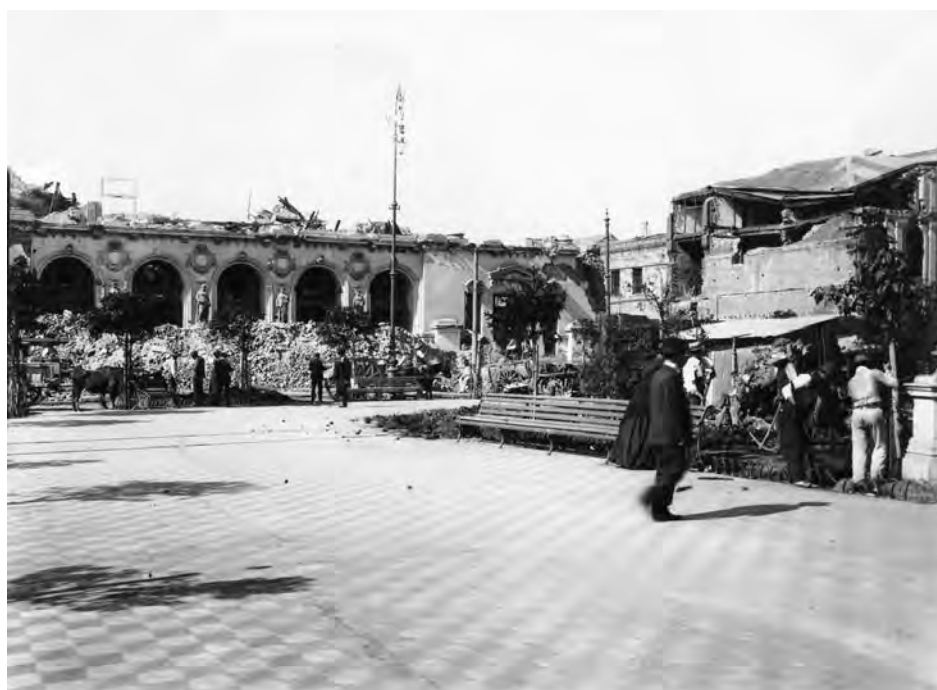
Santiago 1906: Damages after the earthquake of 16.8.1906 (Photo: Fritz Sauter)
